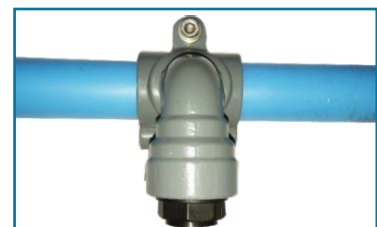
Step 6: Fixing the Droplet on the tube
