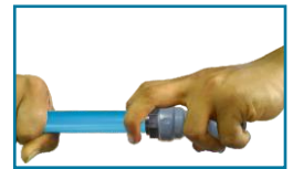
Step 5: Inserting the Tubes into fitting
